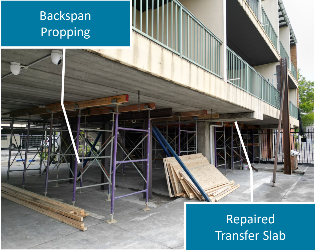
REPAIRED TRANSFER SLAB (WITH PROPPING IN PLACE)
