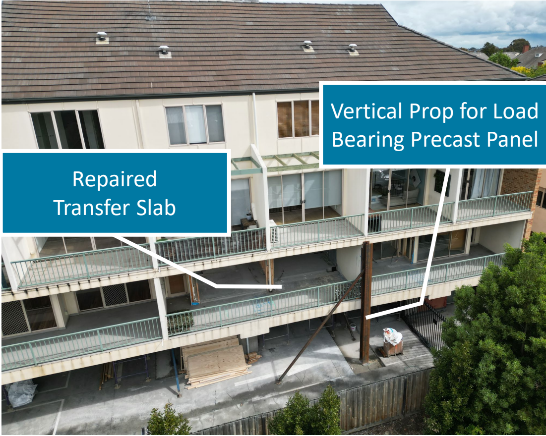
REPAIRED TRANSFER SLAB (WITH PROPPING IN PLACE)
