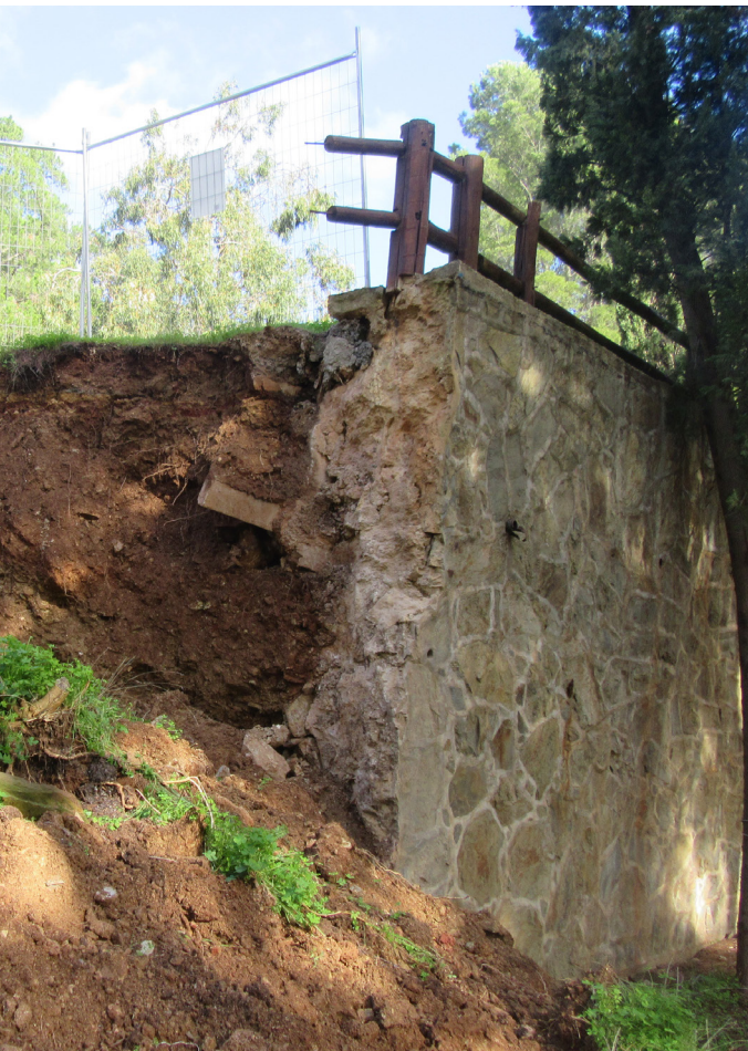
IMAGE: RETAINING WALL FAILURE
