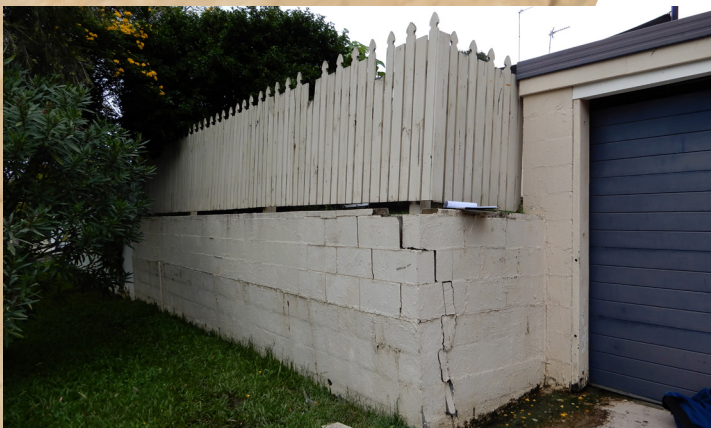
IMAGE: WALL CRACKING
